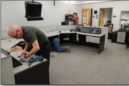
Dismantling the old desks.
