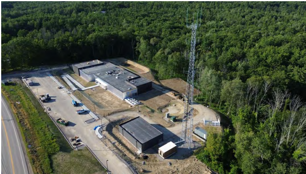
Future home of Lakes Region Mutual Fire Aid Association and new radio tower at 311 Meredith Center Road, Laconia
