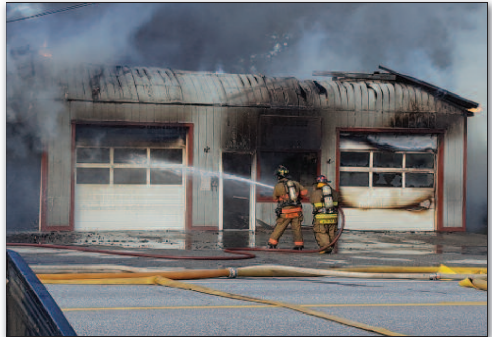
May 17, 2016. Fire at Moses Body Shop on Route 25, Rumney.
